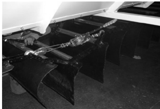
Figure 6 - Using Come-Along To Pull Up Chain Slack
