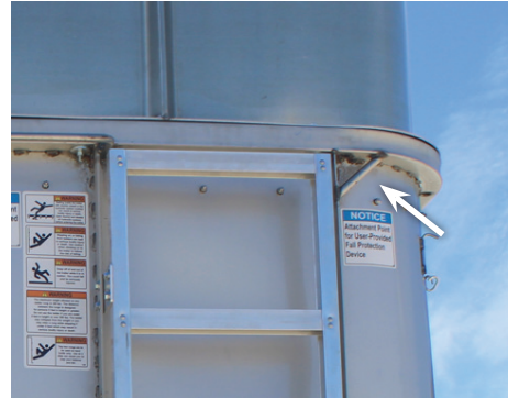
Figure 158 Front Ladder Showing Upper User Fall Protection Device
