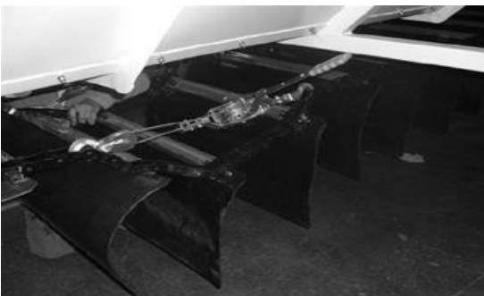
Figure 8 - Using Come-Along to Pull Up Chain Slack
